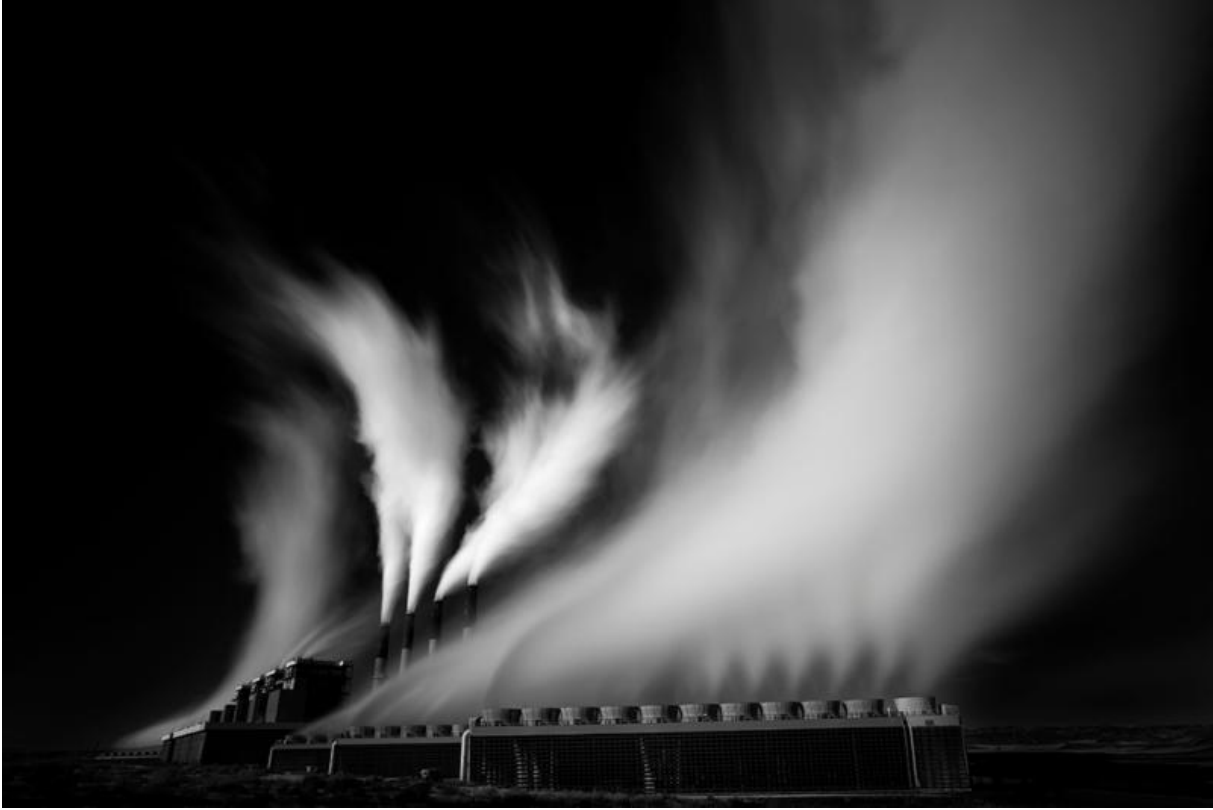
Jim Bridger Power Plant, by Cole Thompson
